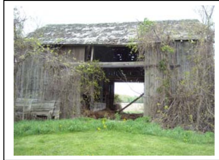
This is the Richard Wright barn being dismantled for materials.
