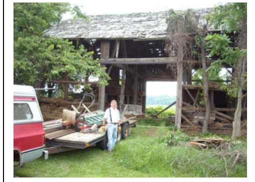
Work in process.
